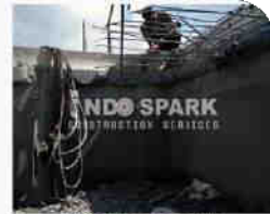
RCC Slab Cutting Work
