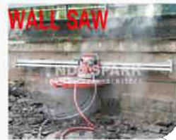
RCC Slab Cutting Work
