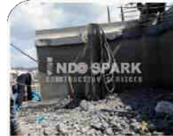
Removing cutouts by the help chainpully
