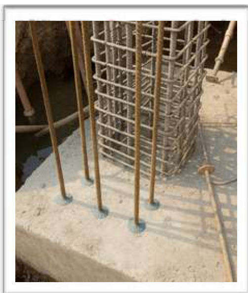
Rebaring for beams & Columns
