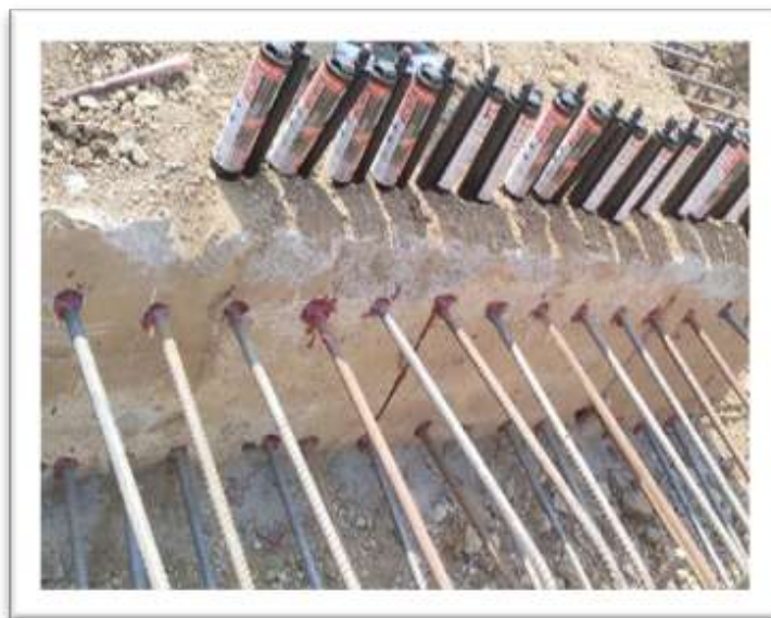
Foundation to column rebaring
