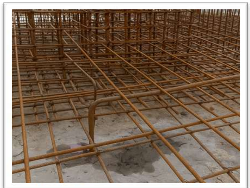
Rebaring for slabs and chajjas
